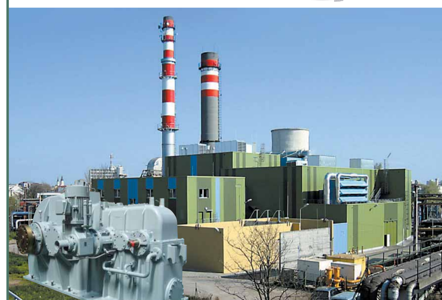
Gas Turbine Generator
